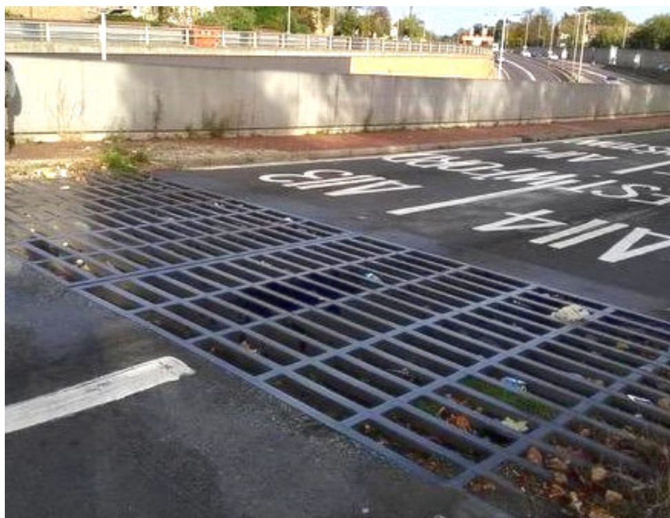
The last reminder of cattle on local roads – a cattle grid still visible at the Green Man roundabout Leytonstone
